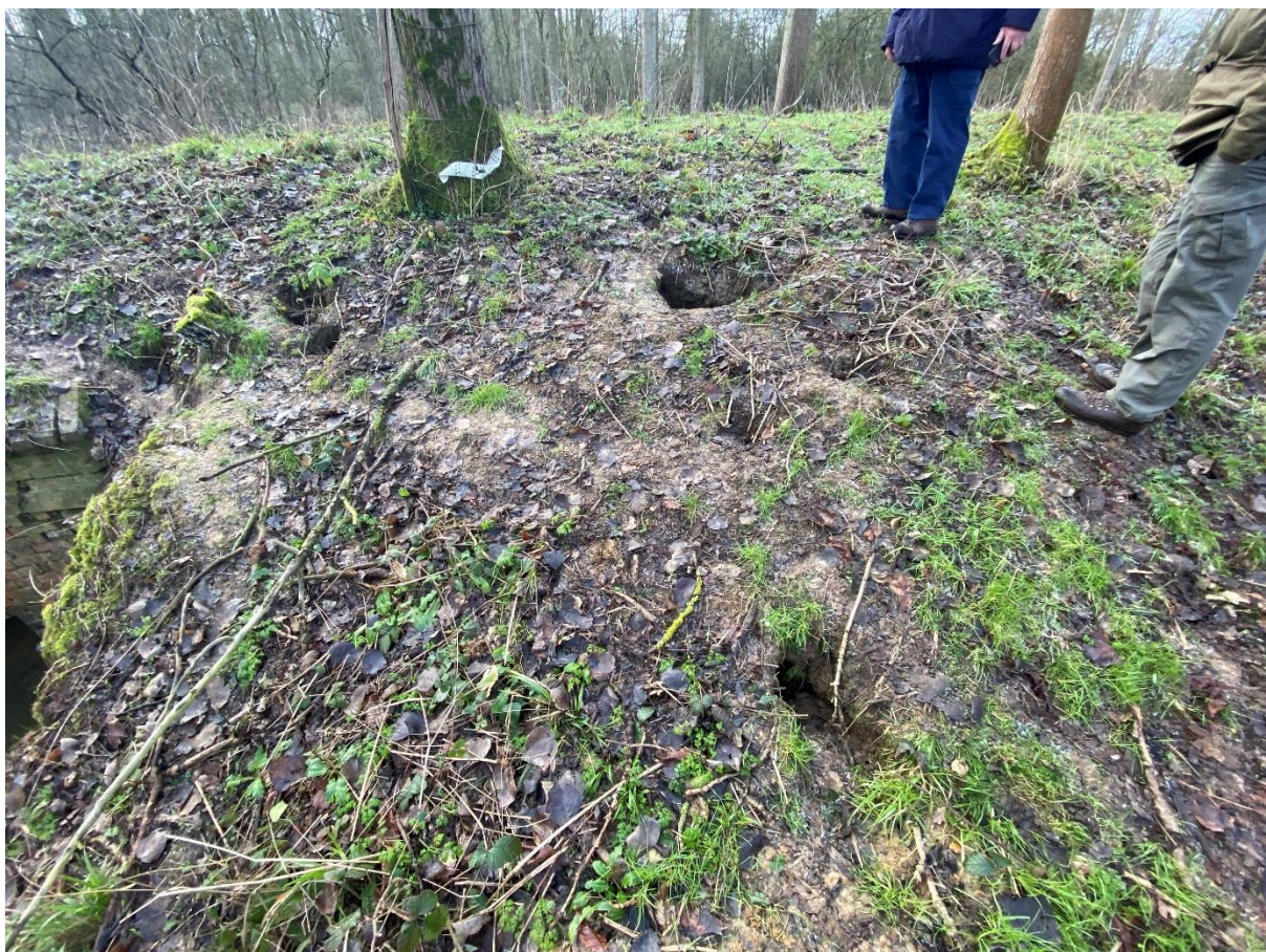
Plate 2 Example of damage to the dam from invasive species, near to one of the culverts.
